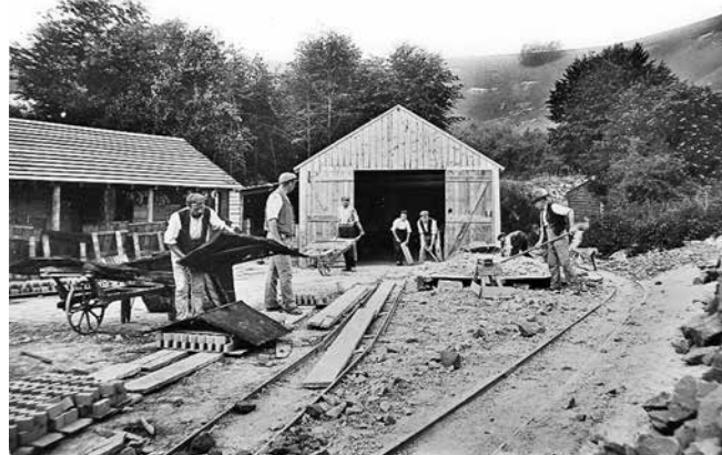
Colley Hill mine hearthstone factory c1910. Completed blocks are seen here set out to dry. Covers to protect them from rain can be seen
